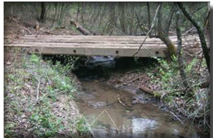
Bridgemats provide a good alternative for temporary stream crossings with minimal impacts to water quality.
