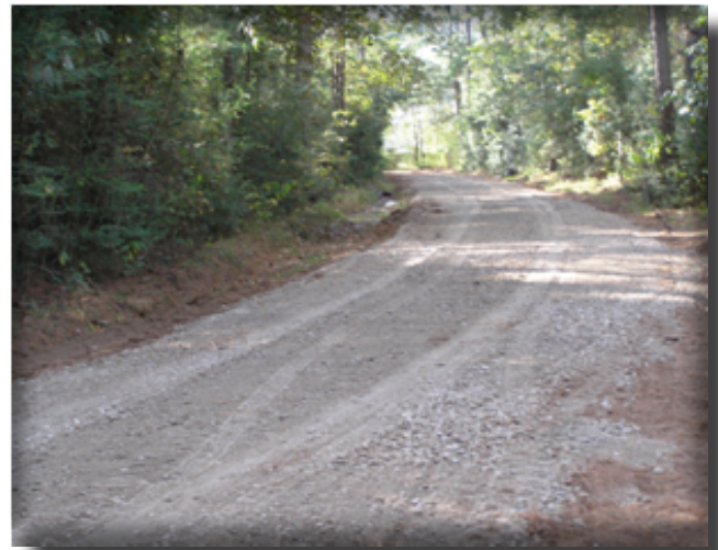
Rock is an excellent choice for roads that remain wet for extended periods of time or for roads with a high erosion potential.
